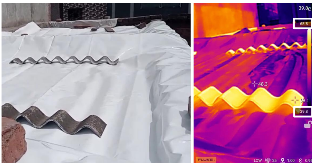
Figure 13 After cool roof installation – roof surface temperature reduced to 48.3 °C, a drop of nearly 20 °C
