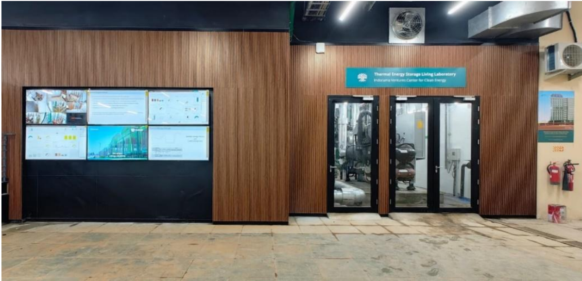
Figure 41 Thermal Energy Storage Lab
