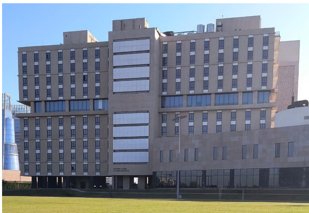
Figure 26 Hostel-1 building (220 rooms) at Plaksha using Thermal Energy Storage for night-time cooling
