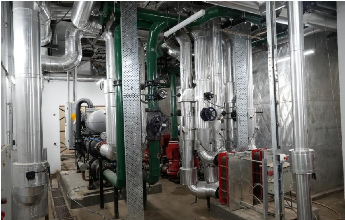
Figure 29 Thermal storage plant piping network
