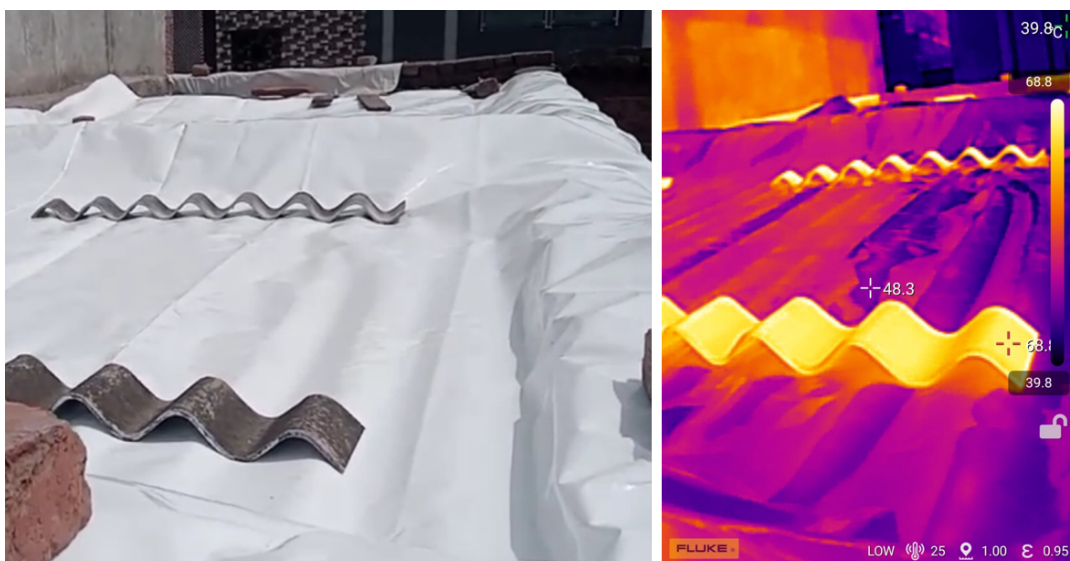
After cool roof installation - roof surface temperature reduced to 48.3 °C, a drop of nearly 20 °C
